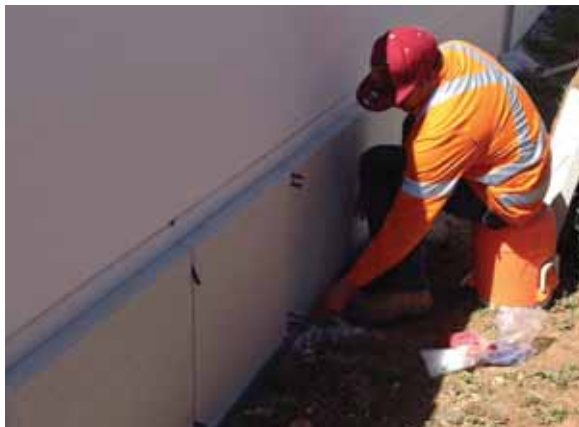
Installing Reapor on site to using flexible, thixotropic adhesive.
