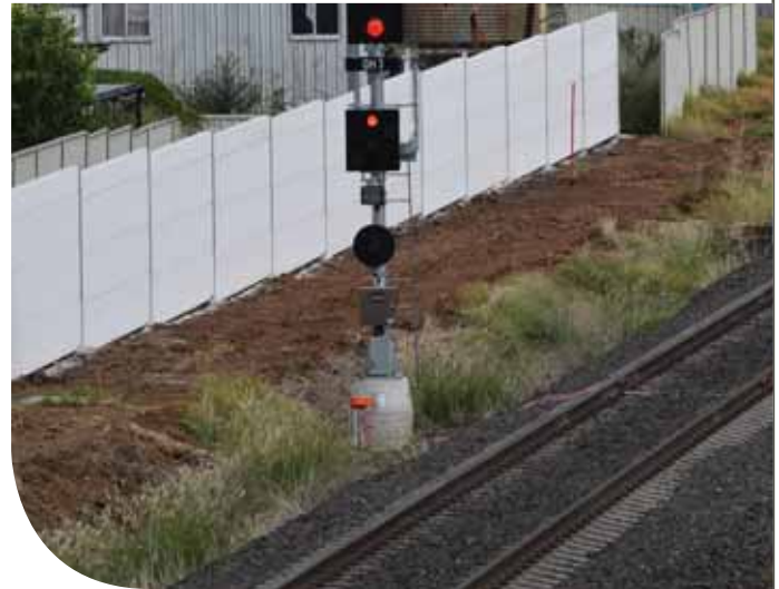
Reapor installed on Noise Wall 1 to protect the Gunnedah community
