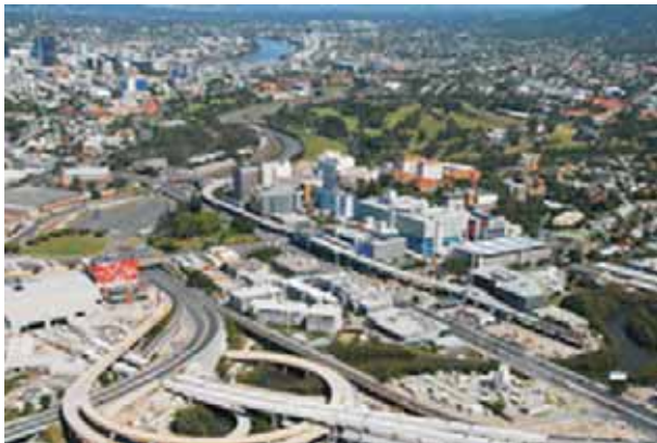
Brisbane North West Road bypass tunnel ventilation shafts
