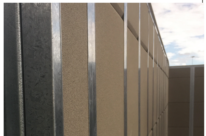
Lightweight Viterolite 300 tiles mechanically fixed to a C-channel frame
