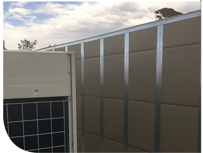
Rooftop HVAC noise containment with high performance wall
