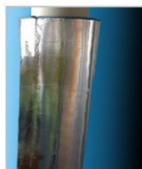
Tape along the longitudinal overlapped length
