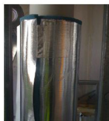
Use small tape patches to secure the wrap and position firmly around the pipe
