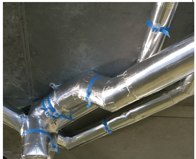
With proper install, the 2053 bathrooms worth of waste water pipes are quieter and particularly effective for problem areas around bends.
